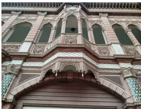
Fig. 5 : Chhajja & Chhajwal (Rampurja Haveli) (Source : Self)
